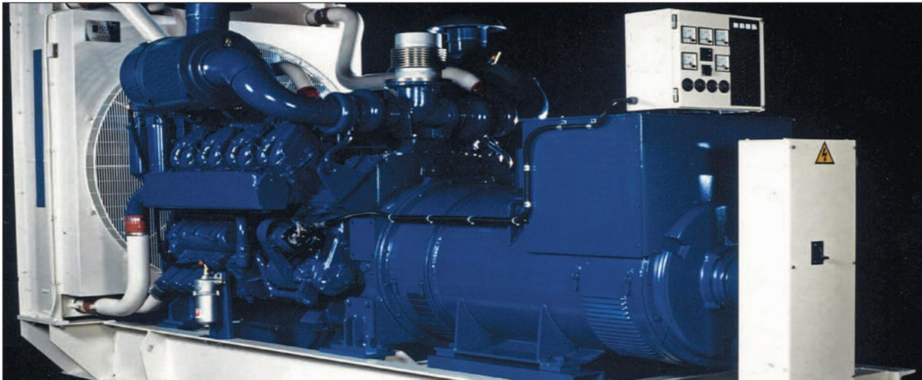
Diesel generator set. Coupling fitted between the engine and alternator.
