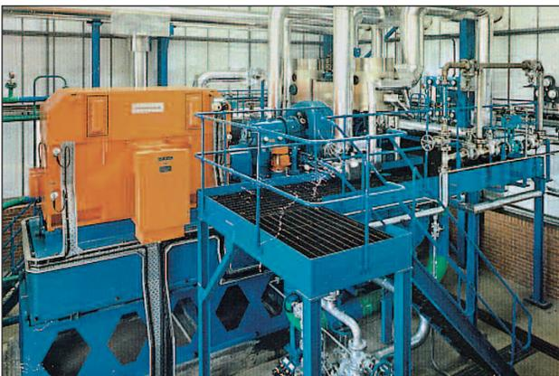
Steam Turbine Generator Set. Coupling fitted between the gearbox and alternator.
